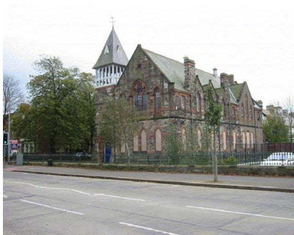
(SOURCE: Architectural Heritage Fund)
